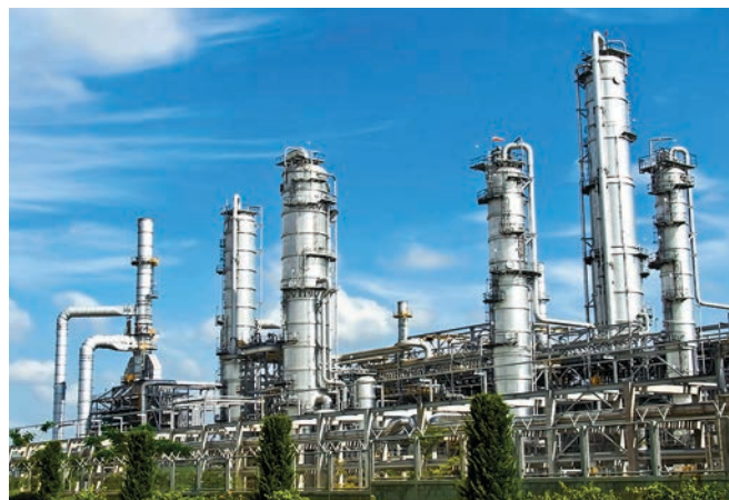
FIG. 1. The potential presence of hazardous toxic, flammable and combustible gases requires refineries to employ a highly reliable safety monitoring system.
