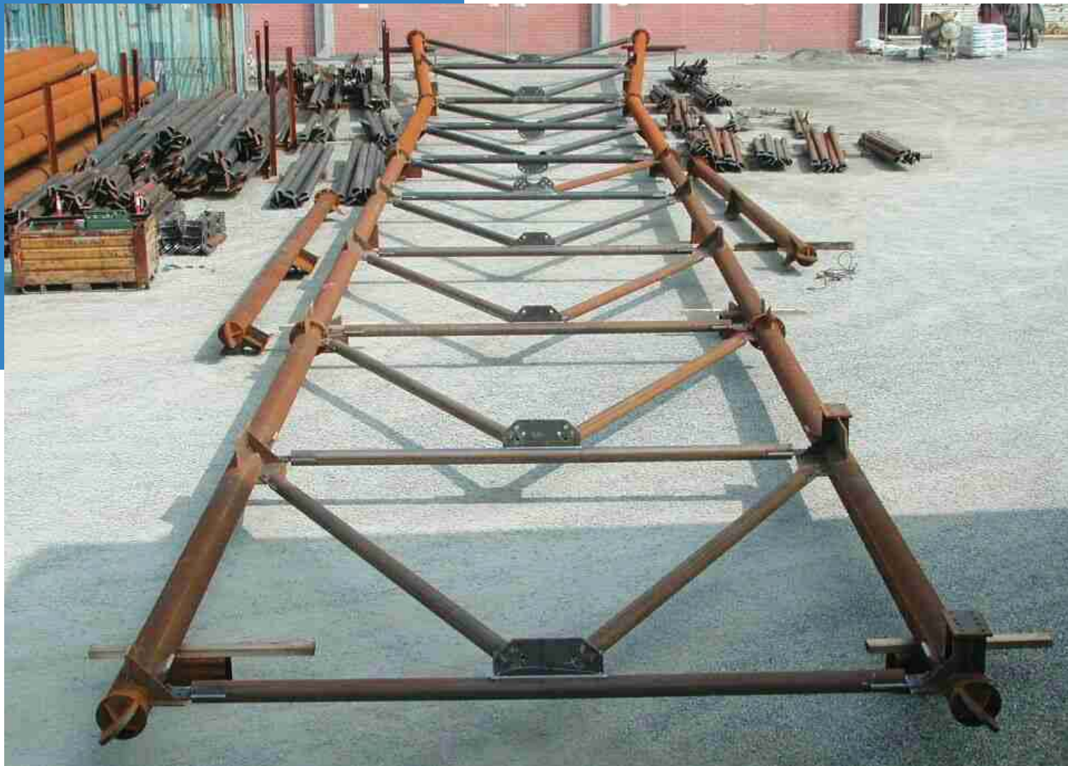
Trial Assembly of Derrick Structure
