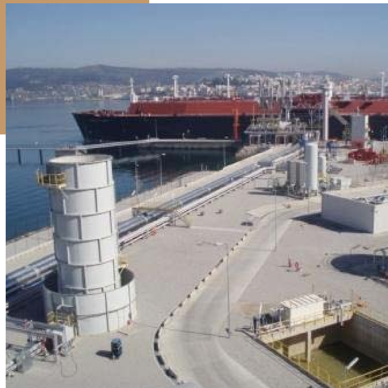
15t/h Enclosed Ground Flare Mugardos, Spain
